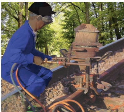
Figure 3.11 Thermit process for joining railway tracks
