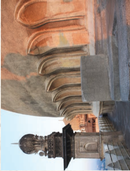
Drum of the Dome
