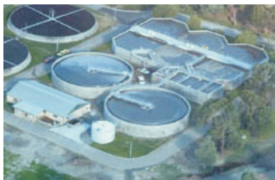
Figure 8.7 An aerial view of a sewage plant
