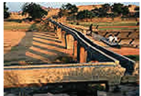
Fig. 7.5 An aqueduct leading into the royal centre
