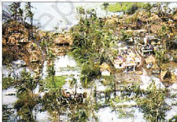
Destruction caused by a cyclone
